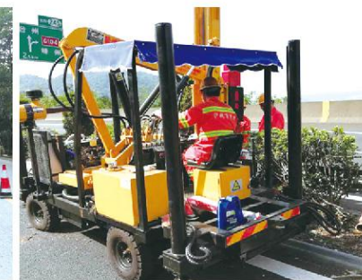
浙江施工 Construction site in Zhejiang
