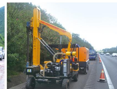
湖南施工 Construction site in Hunan
