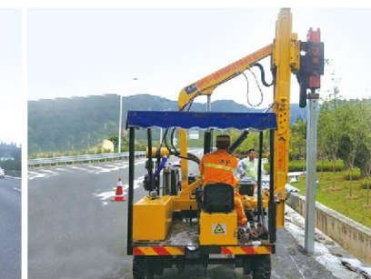
青海施工 Construction site in Qinghai
