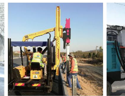
山东施工 Construction site in Shandong
