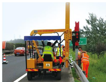
河北施工 Construction site in Hebei
