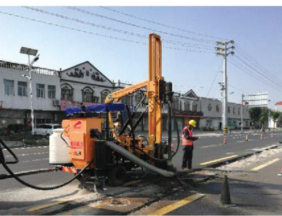
新疆施工 Construction site in Xinjiang
