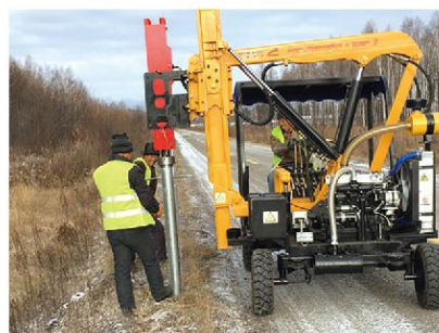
黑龙江施工 Construction site in Heilongjiang
