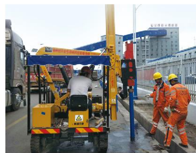
甘肃施工 Construction site in Gansu
