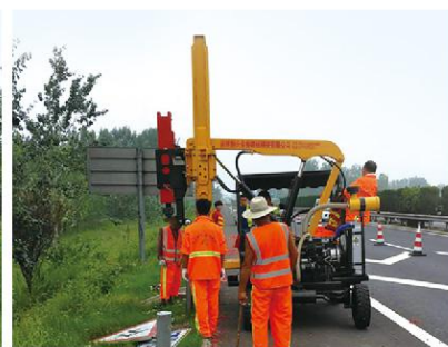
辽宁施工 Construction site in Liaoning
